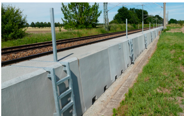
View from the outer side with drainage openings and emergency escape ladders
