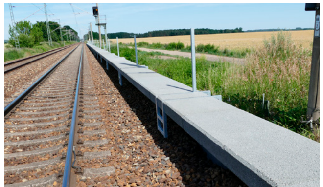
View from the track side, emergency escape ladders positioned every 6 metres
